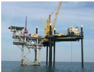
Example of Jack-Up Barge: RAM VII of Aries Marine Corp.
